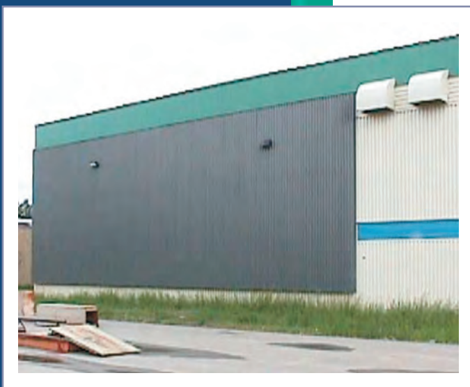
Solar Wall installed on the recreation building in Fort Smith.
