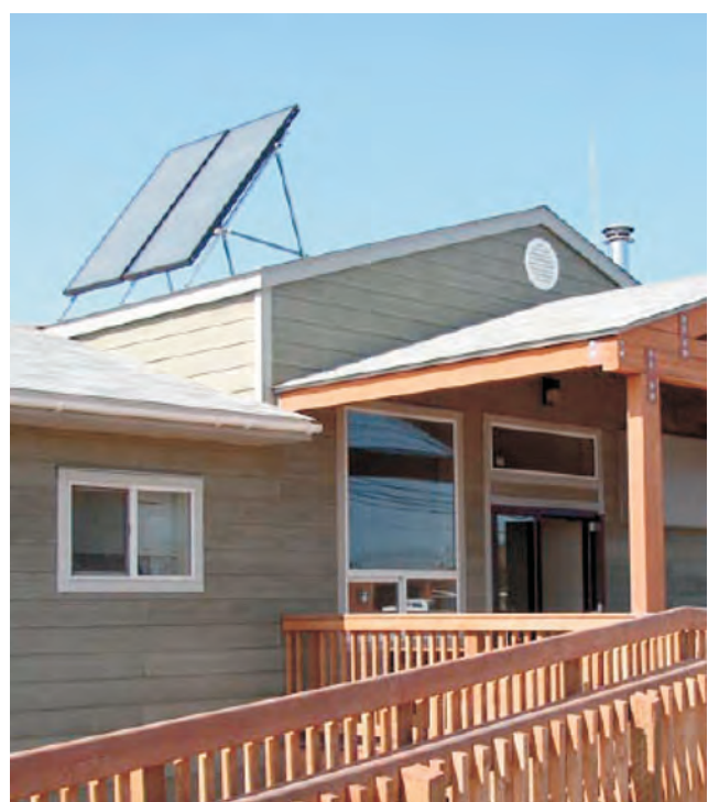
Solar Water Heating on the Elders' building in Whati.
